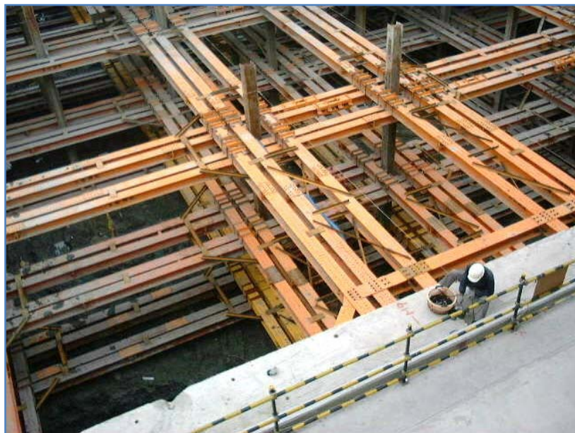
塔樓-第三階開挖-支撐 Tower-3rd Excavation/Strutting
