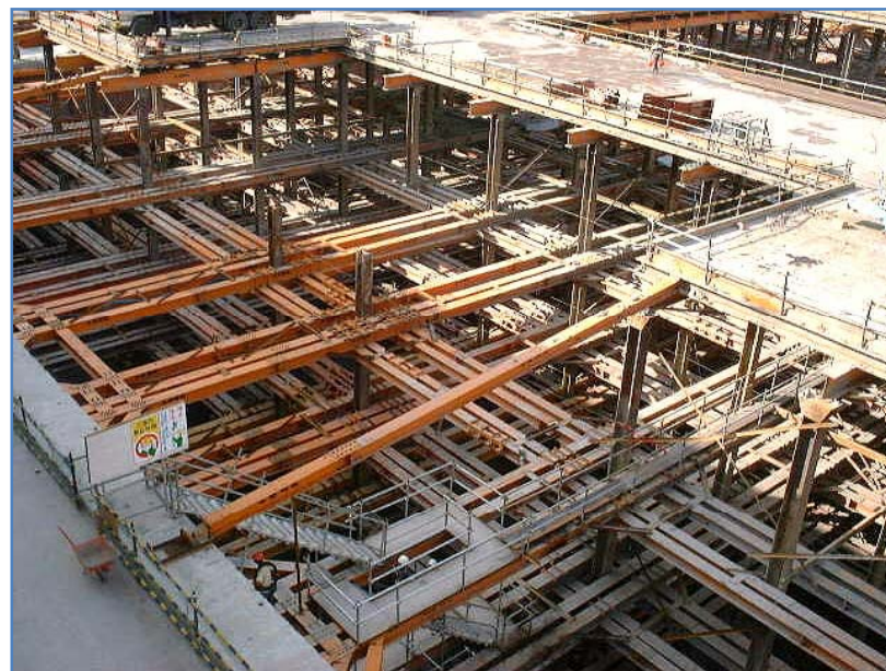
塔樓-第三階開挖-支撐 Tower-3rd Excavation/Strutting
