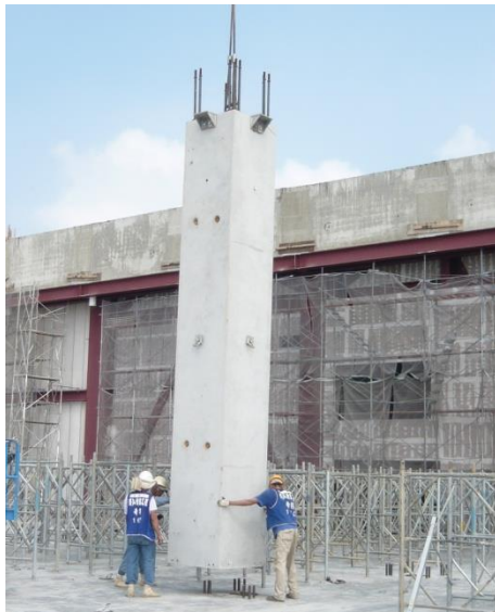
Angel Seating on the top of columns for Girders 預鑄大梁臨時 用之柱頭角鋼
