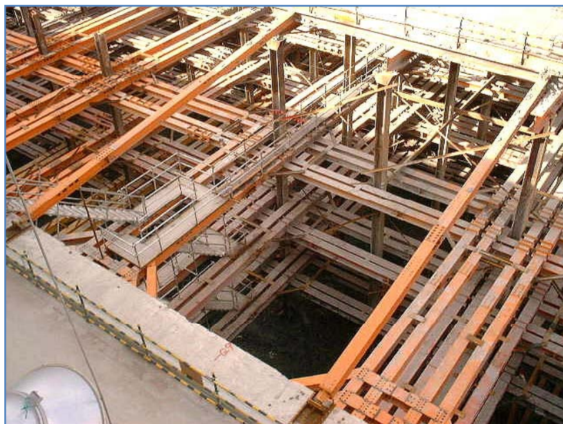
塔樓-第三階開挖-支撐 Tower-3rd Excavation/Strutting
